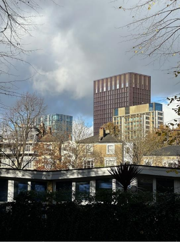
View from Pemberton Gardens in the St John's Grove Conservation Area
