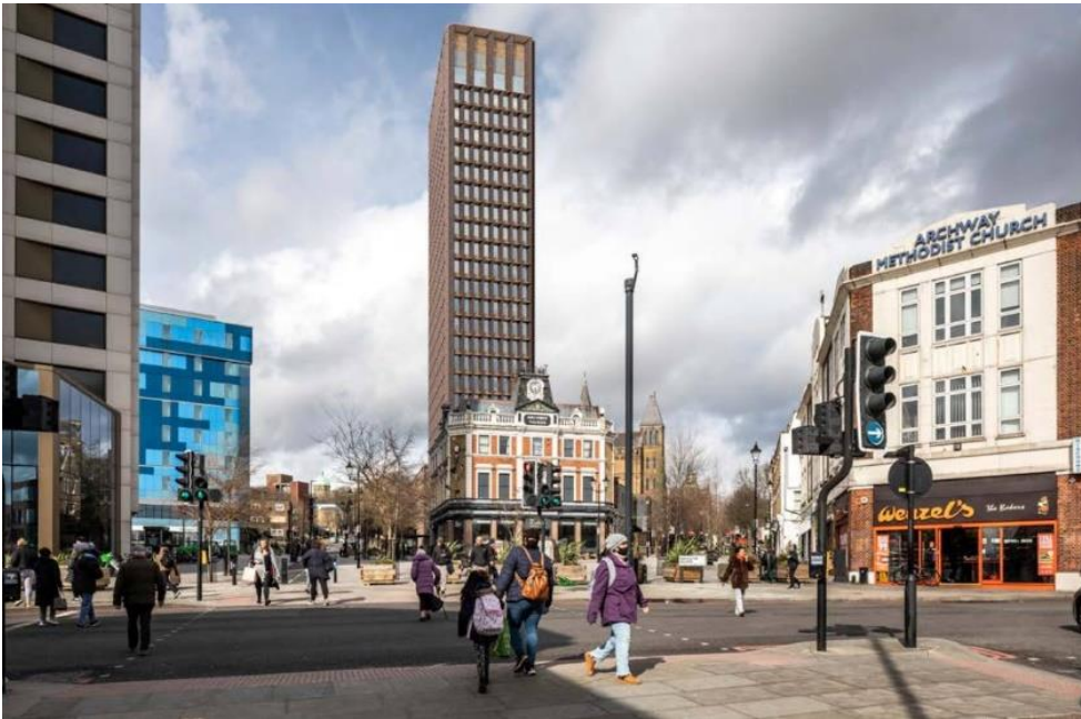
View of locally listed Archway Tavern in the St John's Grove Conservation Area (image provided by Seven Capital)
