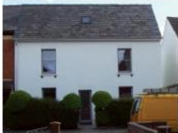
Front elevation post-retrofit
